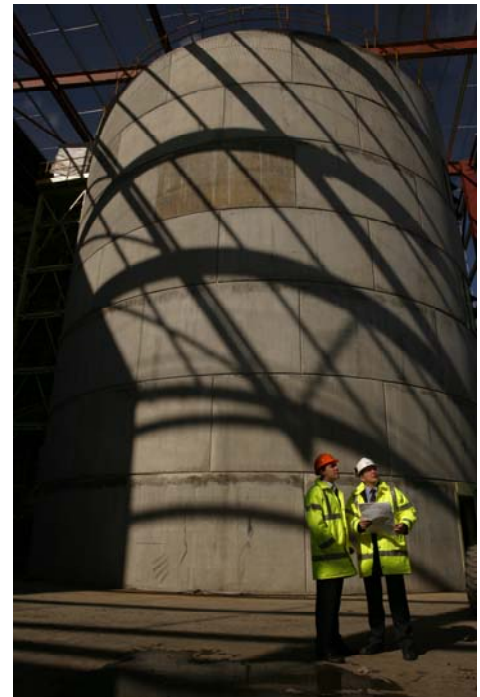
Parc tower 3 during construction
