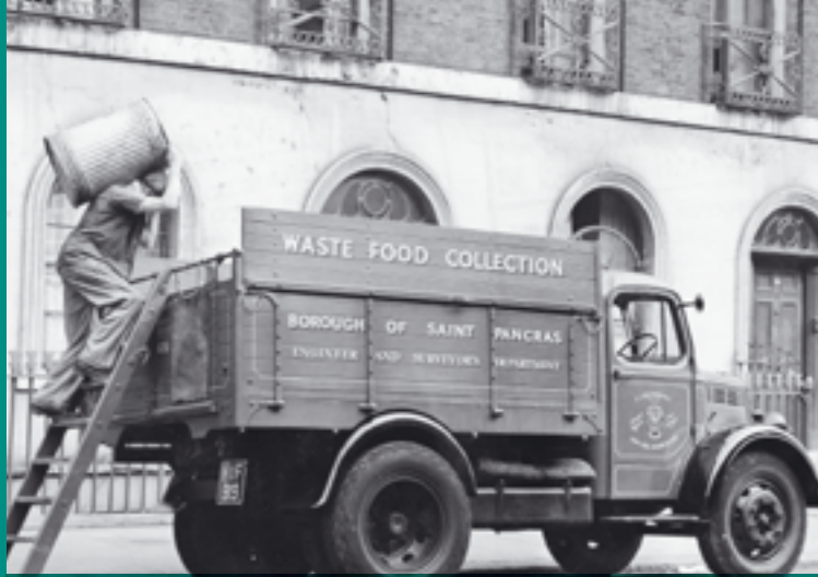
1 - 1948 picture of a Bedford tipper lorry operated by St Pancras Borough Council, collecting food waste for pig feed. A hard climb to empty the 'pig swill' bin.
