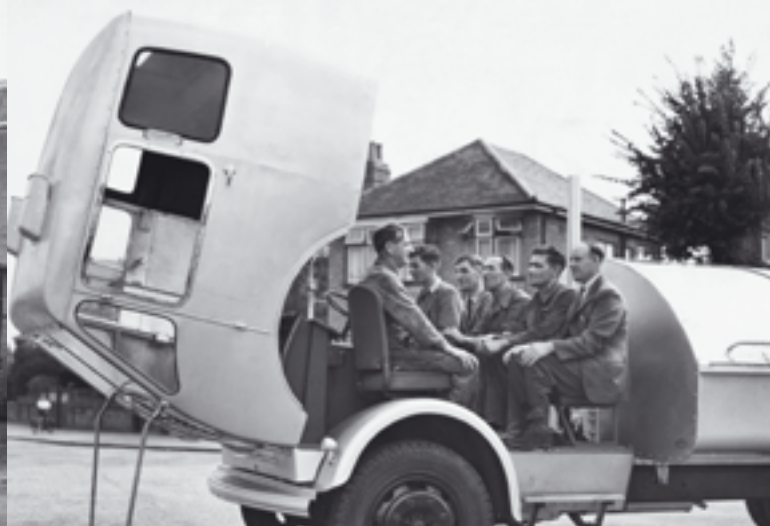
8 - Late 1950s Bedford sideloader – demonstrating the comfortable forward-tilting cab.
